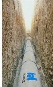
← Sanitary sewer pipe made with composites.
