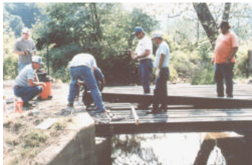
Ü Graphite composite bridge over Toms Creek in Blacksburg, VA.
